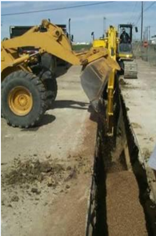
Installation of EHC PRB
